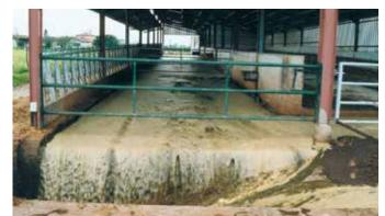
Liquid fraction re-used for flushing
